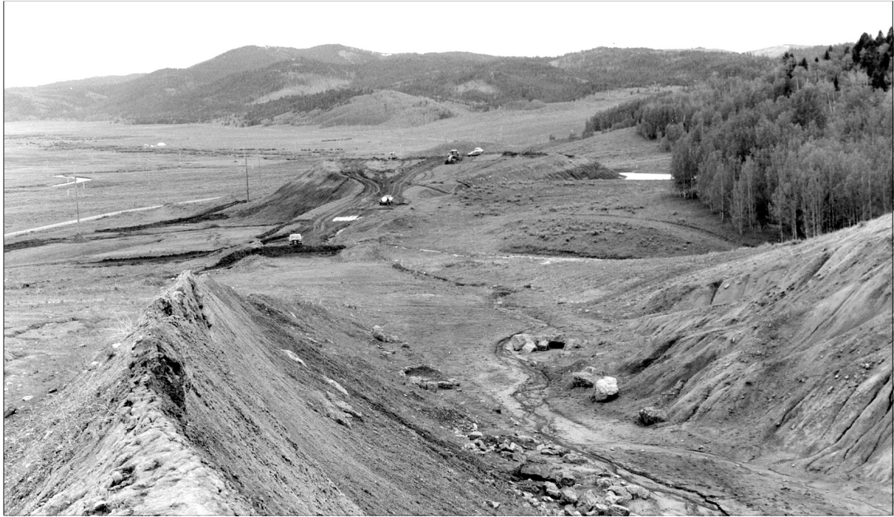
Figure 179. Reshaping Lanes Creek Mine dump by the J. R. Simplot Company, June 8, 1998. Photo by the author.
